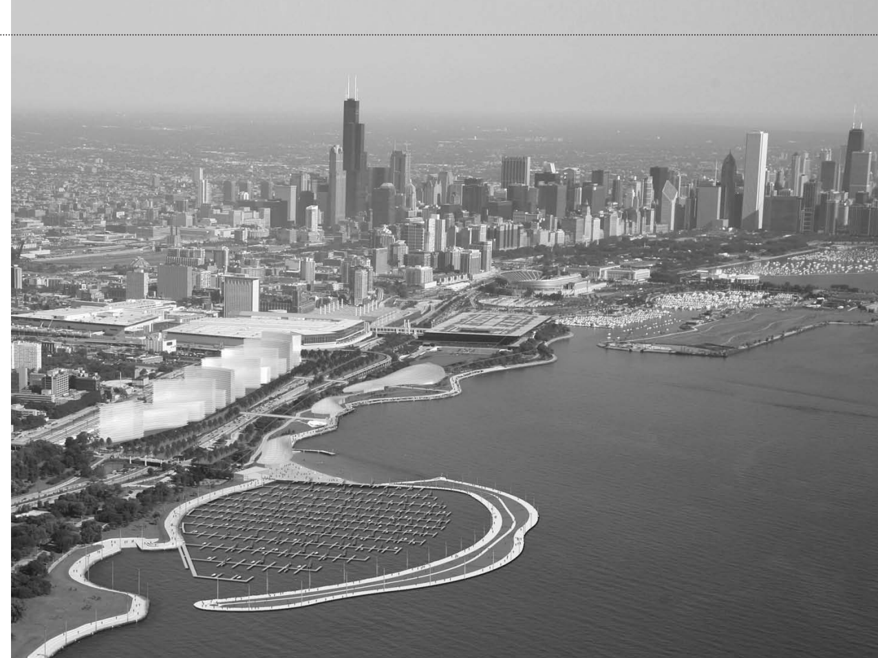
THIS CONCEPTUAL DRAWING OF THE PROPOSED OLYMPIC VILLAGE, COURTESY OF CHICAGO 2016, IS NOT A FINAL DESIGN.
