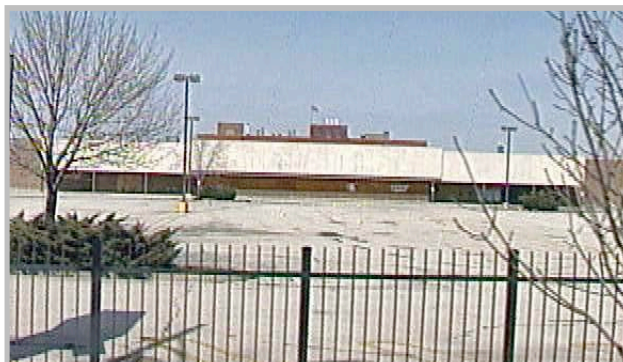
Chicago, IL 1422 W 47th-3rd Ward This former Jewel cannot operate as a supermarket or pharmacy exceeding 20,000 square feet until March 2022.
