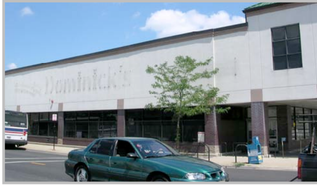
Chicago, IL 3649 N. Central-38th ward This former Dominick's has a restrictive covenant that 'runs with the land'; it can never be occupied by a supermarket or grocery store.
