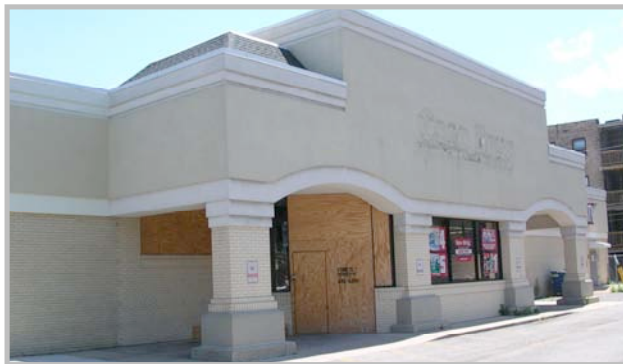
Chicago, IL 1425 W. Morse-49th ward This former Osco Drug cannot operate as a drugstore until August 2024; it has been subdivided and a portion of the former Osco is being leased to Family Dollar.
