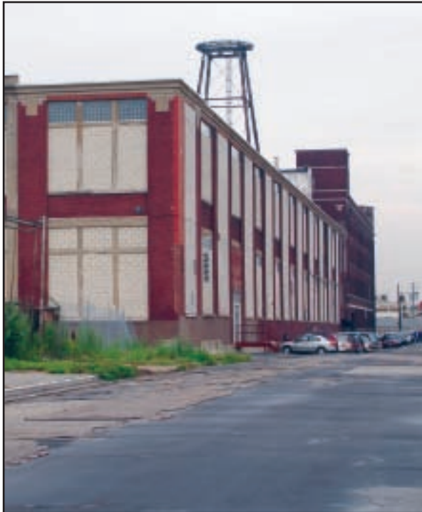
The back section of the otherwise landmarked Western Shade Cloth building (seen in the distance). The panel saw potential for this space, including much-needed parking, large public gatherings, or multi-use space for the creative industries.
