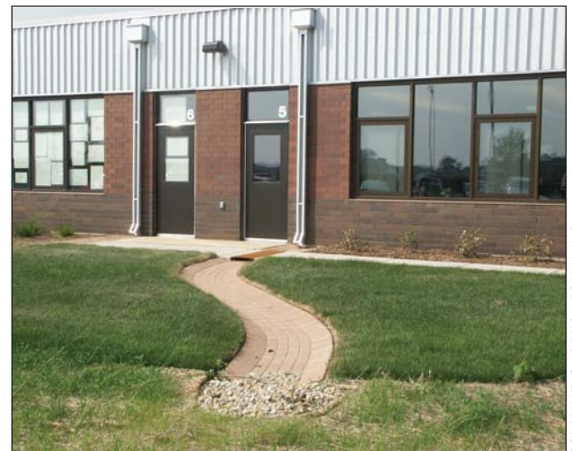
Stormwater can be captured and directed into swales of natural vegetation that will purify and infiltrate the runoff.
