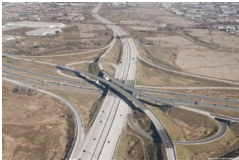
Highway 407 East Extension
