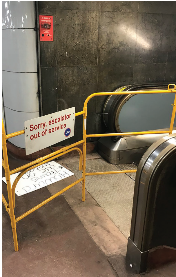
Audrey Wennink @awennink: This escalator at the Monroe El station has been out of service for more than a year
