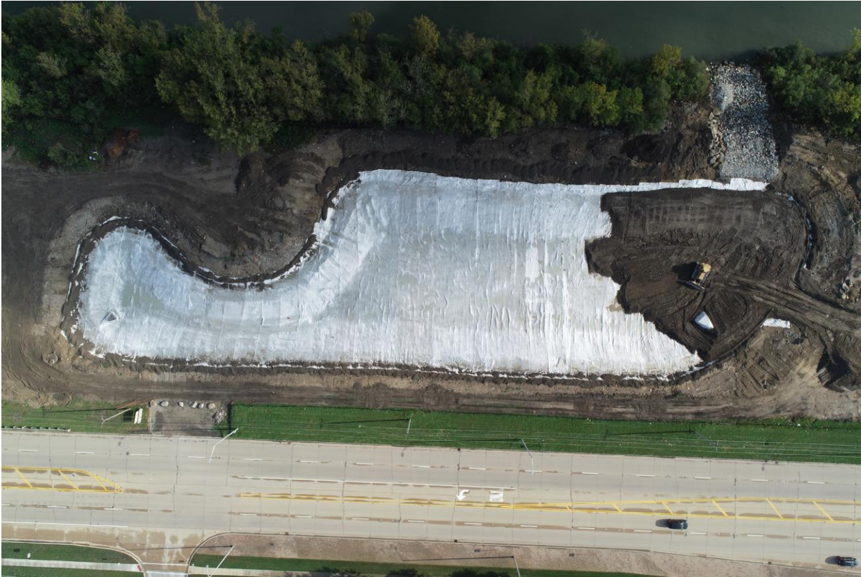
Cal-Sag Detention Basin, Crestwood
