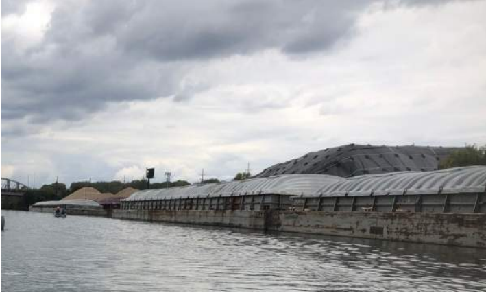
The concrete operation and armored shoreline.
