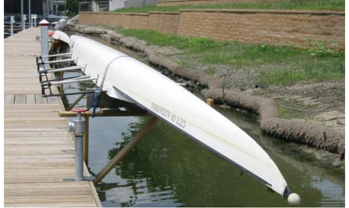
Restored bank and dock.
