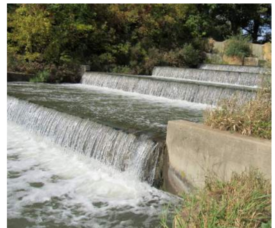
MWRD's SEPA station at SEPA#2. The oxygenated water benefits aquatic life.
