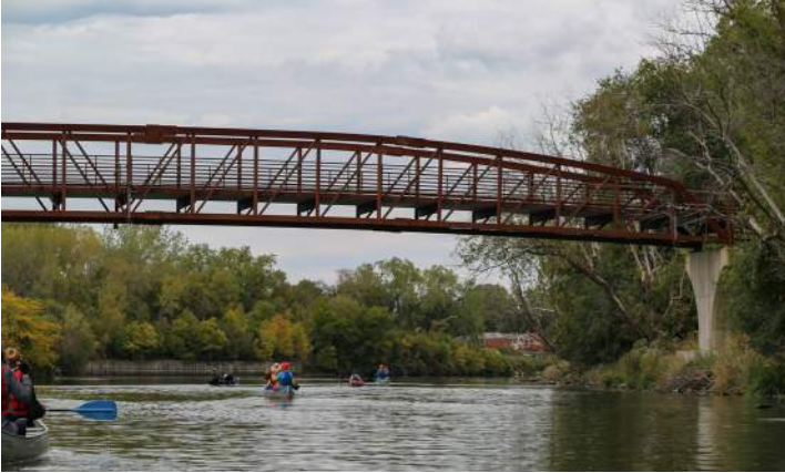
Fay's Point and the Joe Louis Golf Course are connected by the Cal-Sag Trail Bridge.
