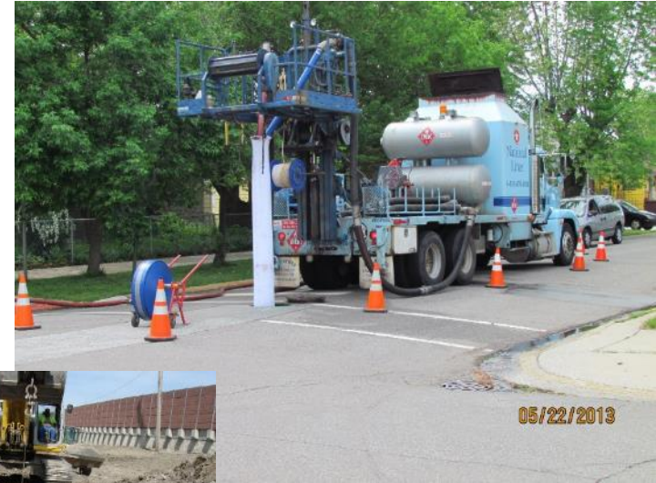
Pipelining operation in East Chicago, IN
