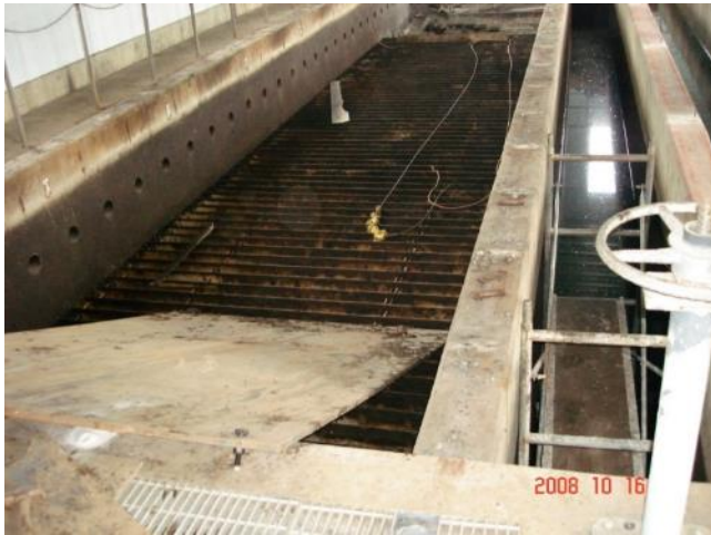
Portage Municipal Water Reclamation Facility
