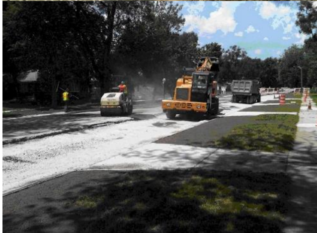
Town of Griffith new storm sewers
