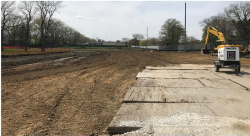
STRIPPING OF TOPSOIL IN PREPARATION FOR EXCAVATION
