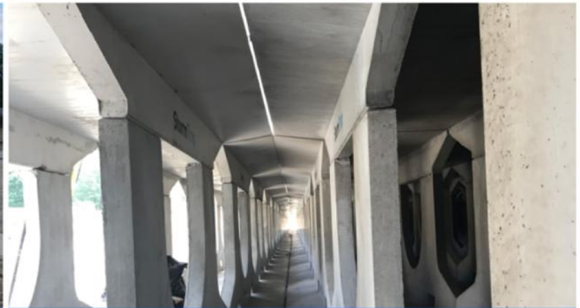
INSTALLED DETENTION VAULT SECTIONS
