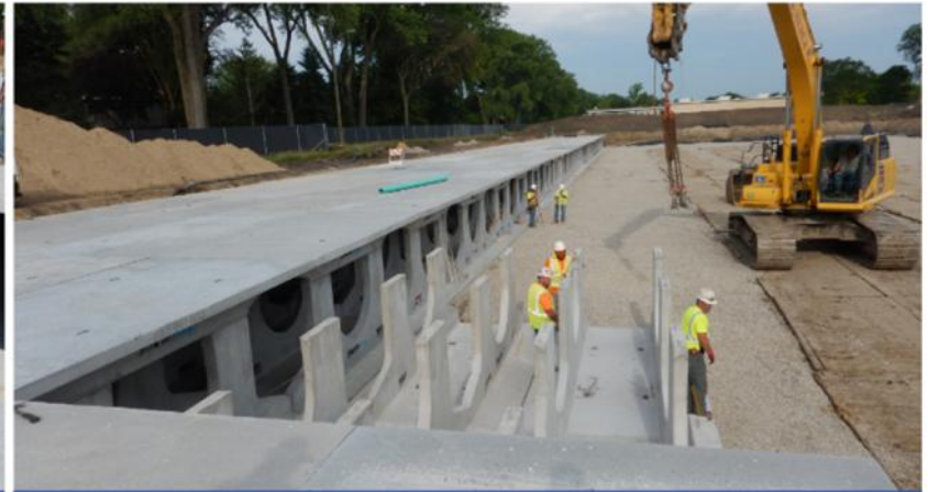
INSTALLING DETENTION VAULT SECTIONS
