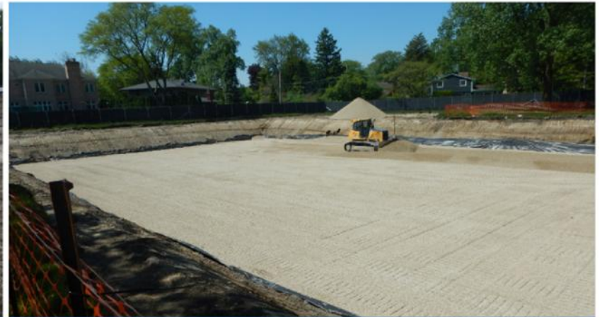
PREPARING BASE FOR DETENTION VAULT
