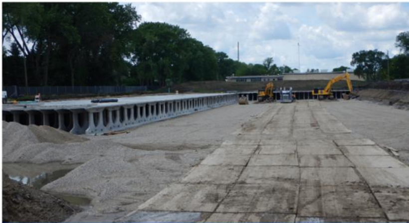
INSTALLING DETENTION VAULT SECTIONS
