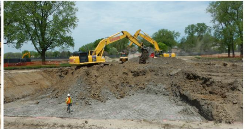
EXCAVATION FOR DETENTION VAULT
