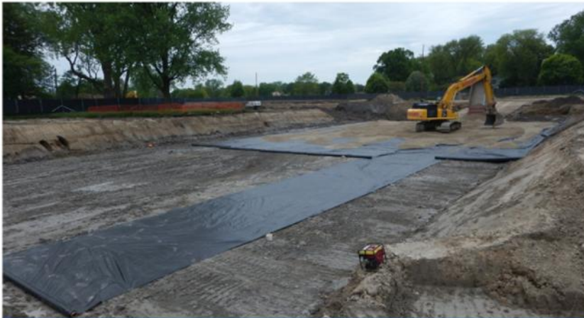
PREPARING BASE FOR DETENTION VAULT
