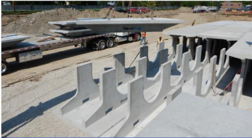
INSTALLING DETENTION VAULT SECTIONS
