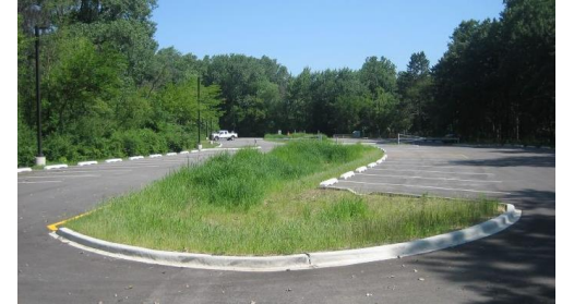
Parking Lot Retrofitted with Bioretention at FPCC Sand Ridge Nature Center (South Holland, IL)
