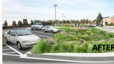
TNC Retrofit of Parking Lot at Sacred Heart Church (Detroit, MI)
