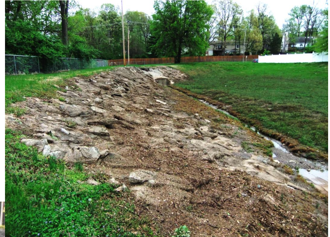
Concrete reinforced banks
