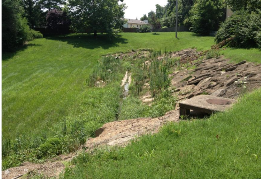
Concrete low flow channels
