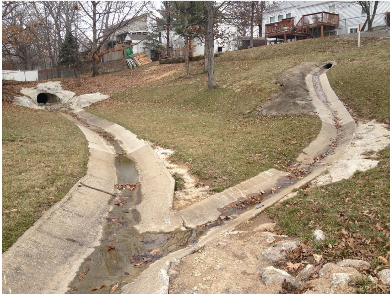
Concrete low flow channels
