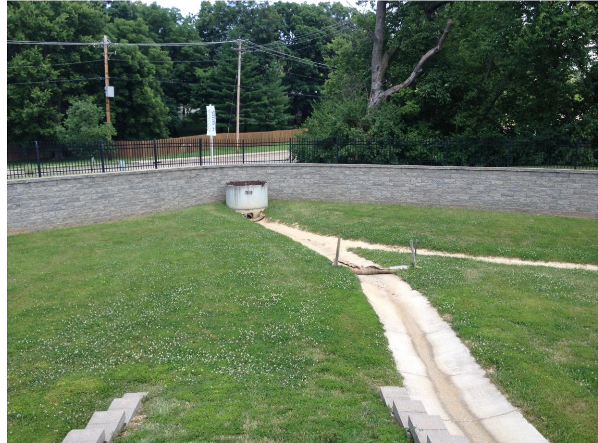
Concrete low flow channels
