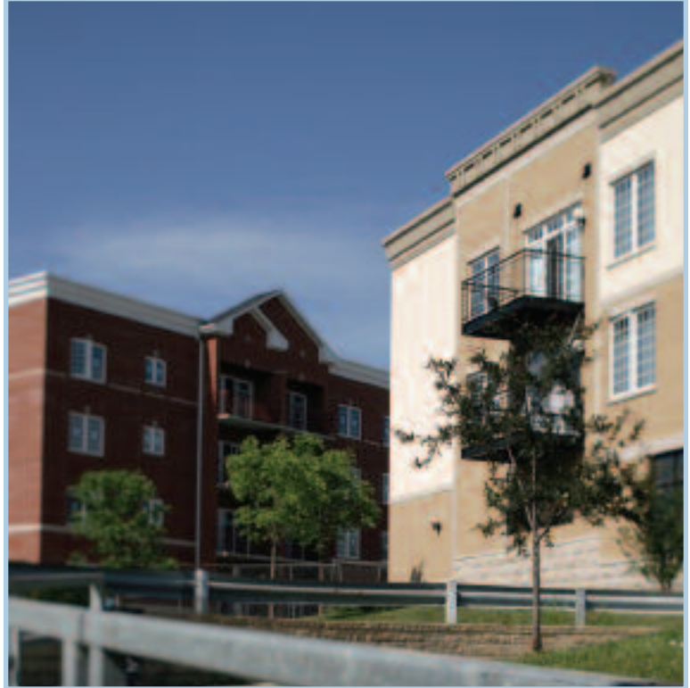
This development in Rolling Meadows includes 30 units (out of 154 total) for low to moderate income seniors. The village is using tax increment financing to cover the gap between market and affordable selling prices.
