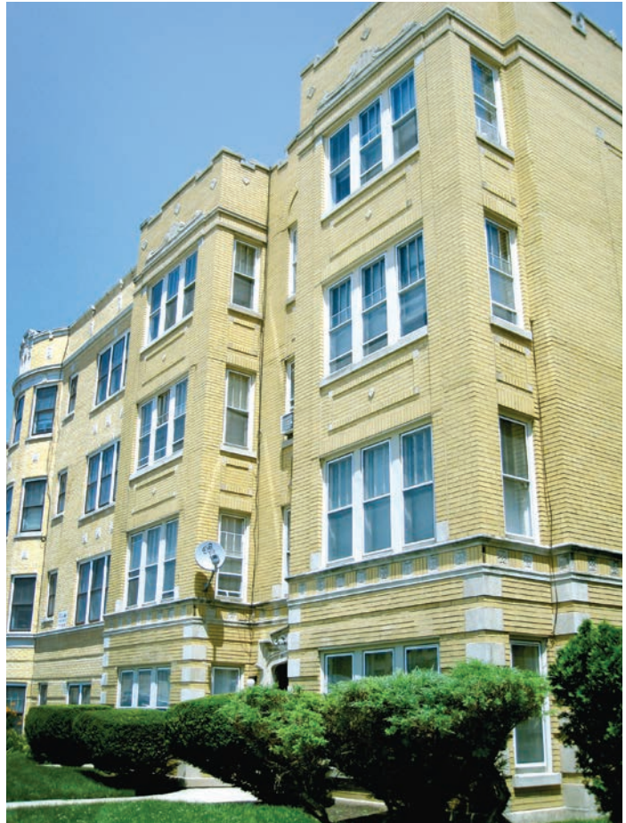
Multifamily buildings in Berwyn range from 2- and 3-flats to larger buildings like this one.
