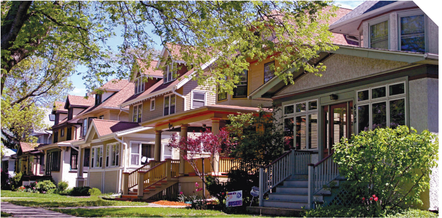
The village includes many blocks of small-lot single family housing like this one.
