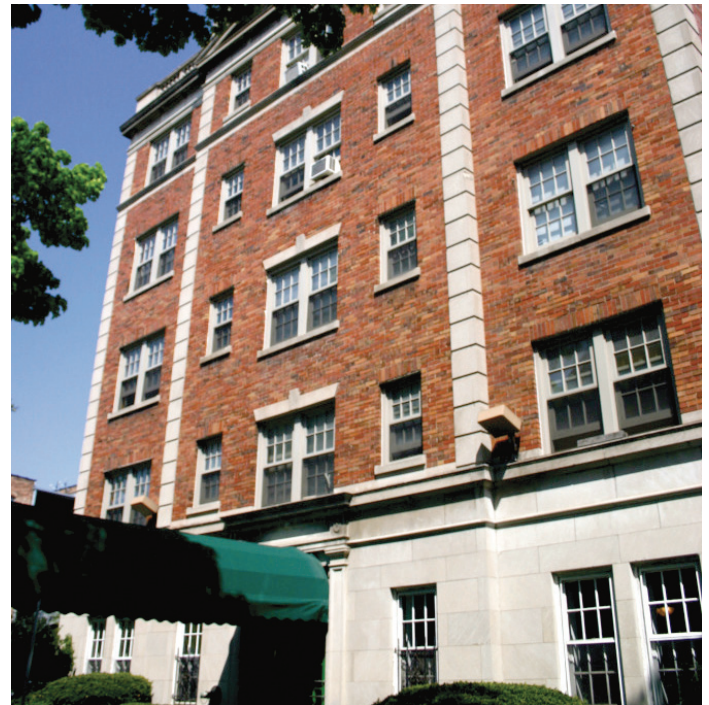
An example of a 1920's apartment building that has been recently rehabilitated to provide updated rental housing while still maintaining historic charm.
