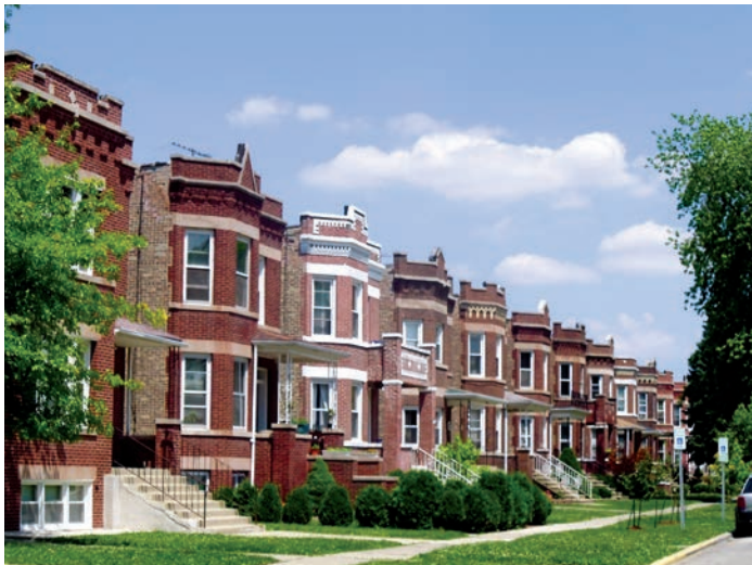
Like many older municipalities in the region, Berwyn has a substantial stock of 2- and 3-flat brick walk up buildings.
