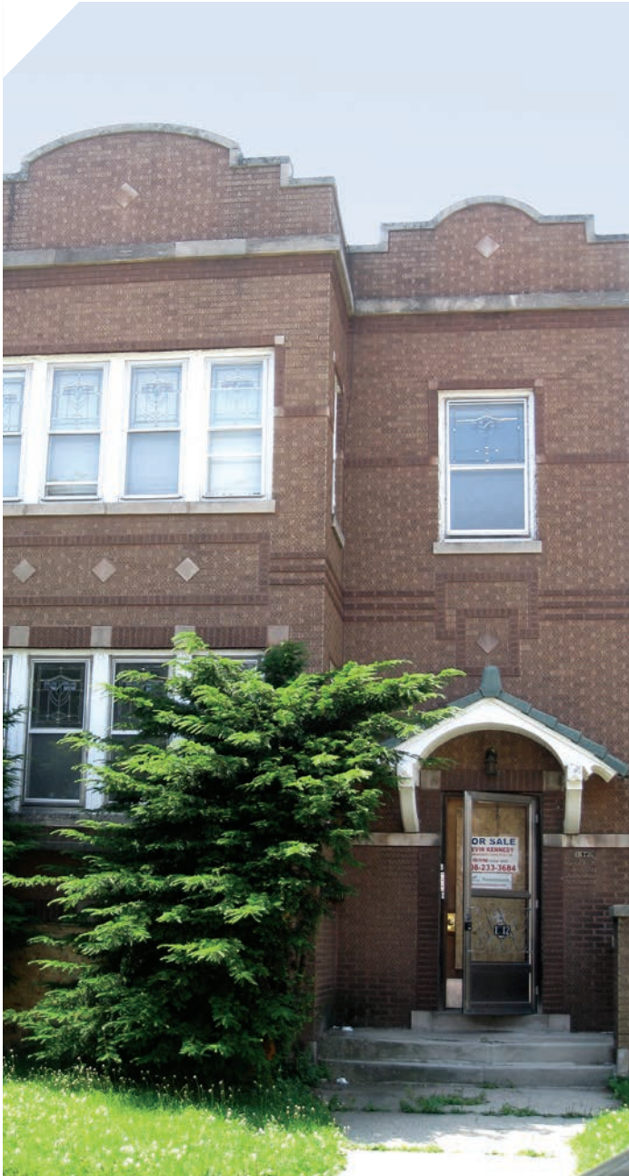
Foreclosure filings have increased especially in small multifamily buildings.
