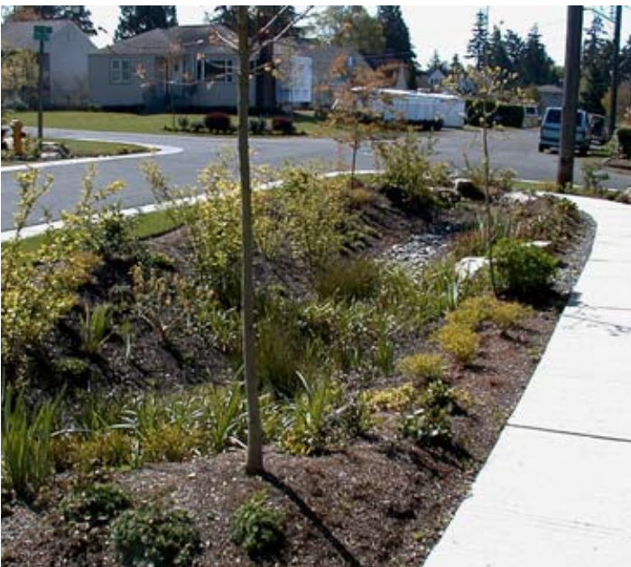
Street swales like this one above help to reduce the amount of stormwater runoff into the public sewer system.
