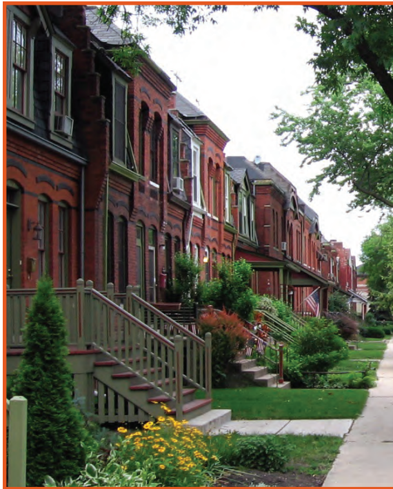
Originally built for employees of the Pullman Palace Car Company, these preserved homes on Chicago's south side continue to be moderately priced.
