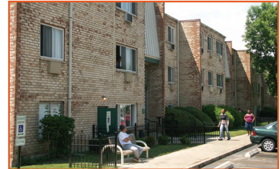
Addison's affordable College Park Apartments were once an eyesore. However, use of LIHTCs and other financial incentives led to rehabilitation and preservation.
