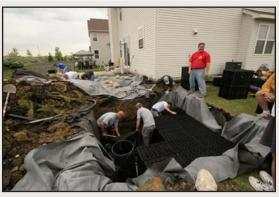
Aquascape employees installing a 1,000 gallon rainwater harvesting system at a home in Oswego, Ill. This water will be used for outdoor irrigation but its not currently tapped for non-potable uses such as flushing toilets.
