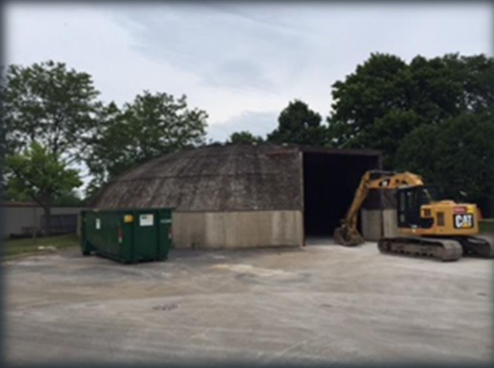
Old Salt Storage Facility – 1,850 Ton Capacity
