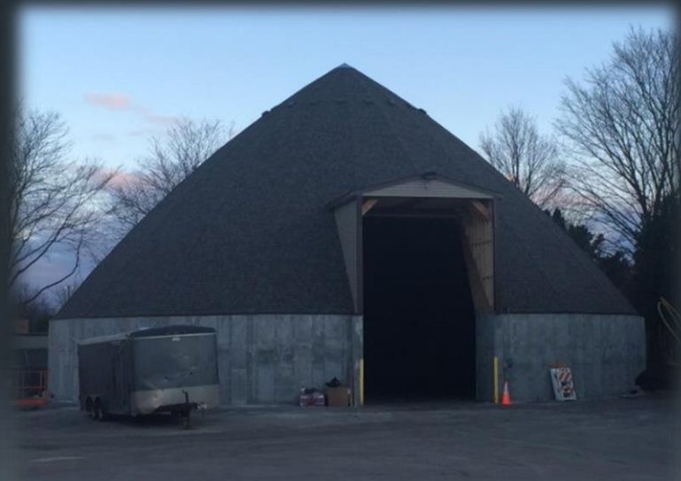
New Salt Storage Facility – 3,700 Ton Capacity
