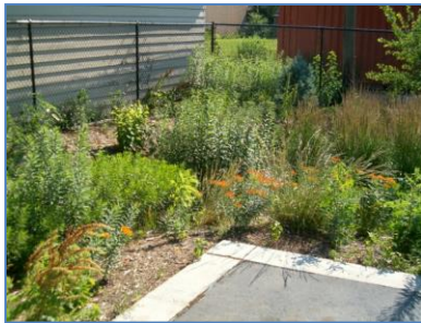
Induced Stormwater Infiltration
