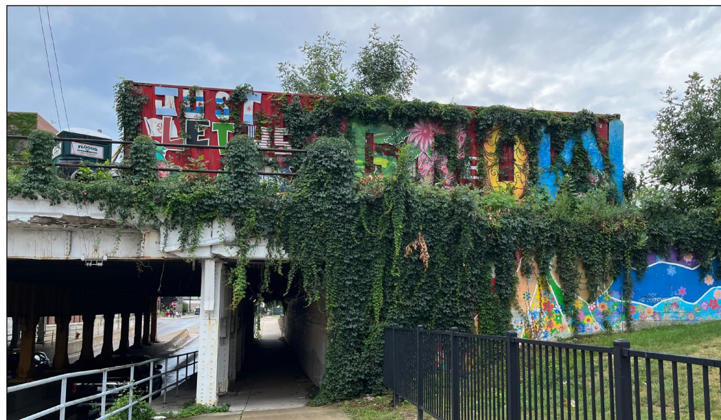
Figure 4. Viaduct Under Rail Line on South Homan Avenue, North Lawndale
