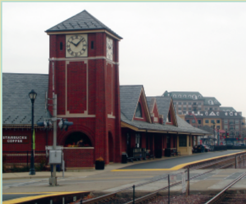
The TOD around Palatine, Ill.'s, Metra station includes mixed-use retail and housing (under construction in the background), office space, entertainment, and both street-level and structured parking.
