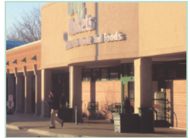
This neighborhood center, at the intersection of 55th Street and Lake Park Boulevard in Hyde Park, is anchored by a Walgreens, ACE Hardware, and a locally owned supermarket.
