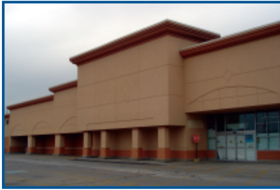
This “white elephant” is in a northwestern suburb; many retail corridors have one. Fortunately, there are proactive strategies to avoid them.
