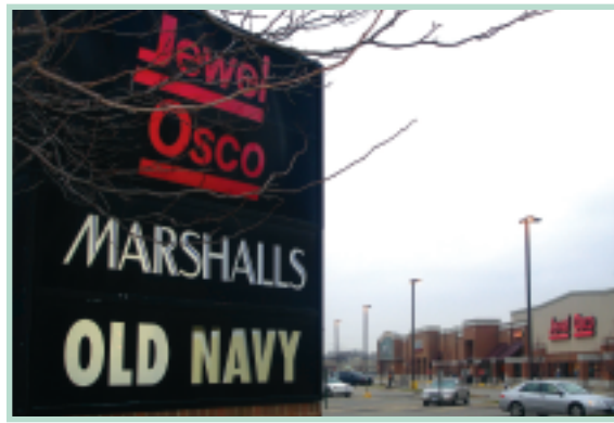
In Skokie, Ill., a former Venture was rebuilt into a Jewel and Old Navy in the 1990s. By reusing the space, Skokie was able to save itself the expense of demolition.
