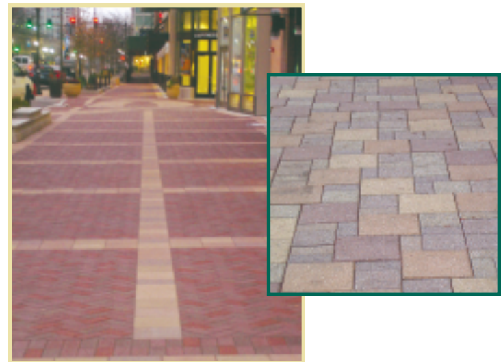
These sidewalks in Evanston, Ill. (left) and Elmhurst, Ill. (right) were upgraded in advance of planned retail development. The attractiveness and durability of these sidewalks can increase the market potential around them.
