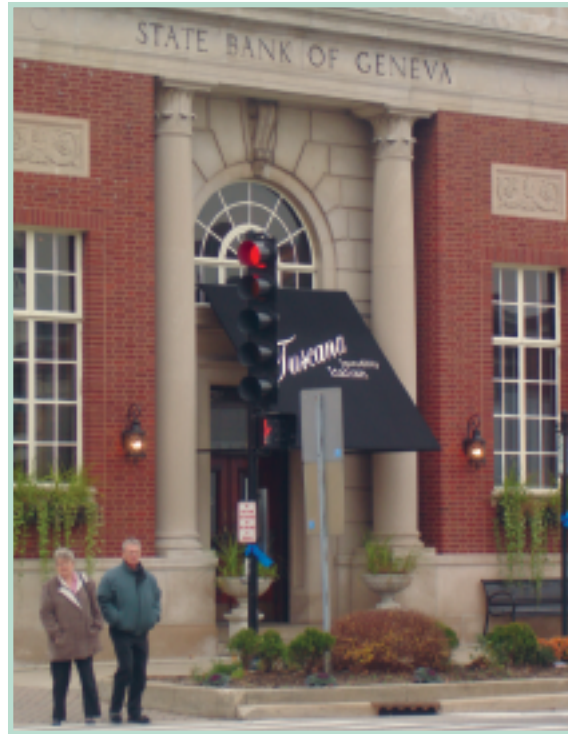
Once the site of the State Bank of Geneva, Tuscana, an Italian restaurant in Geneva, Ill., is a local example of adaptive reuse.
