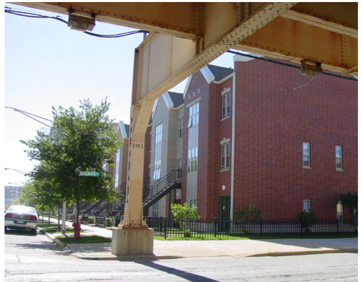
Elevated Green Line tracks above Lake Street
