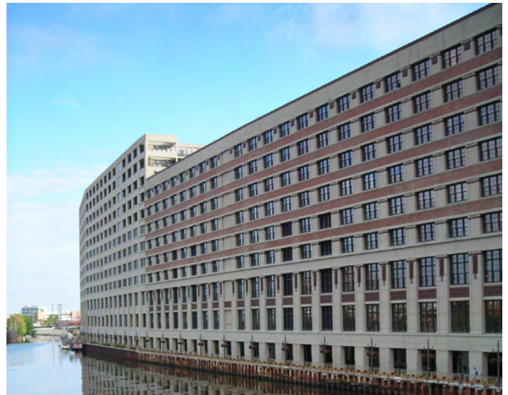
Adaptive re-use at 600 West Chicago Avenue lines the North Branch of the Chicago River.
