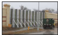
These removable flood wall panels are installed with posts and slots in permanent structures.
