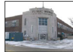
The first floor of the Public Works building continues to undergo reconstruction and rehabilitation.
