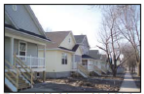
These new single-family homes are being built in the Oak Hill Neighborhood.
