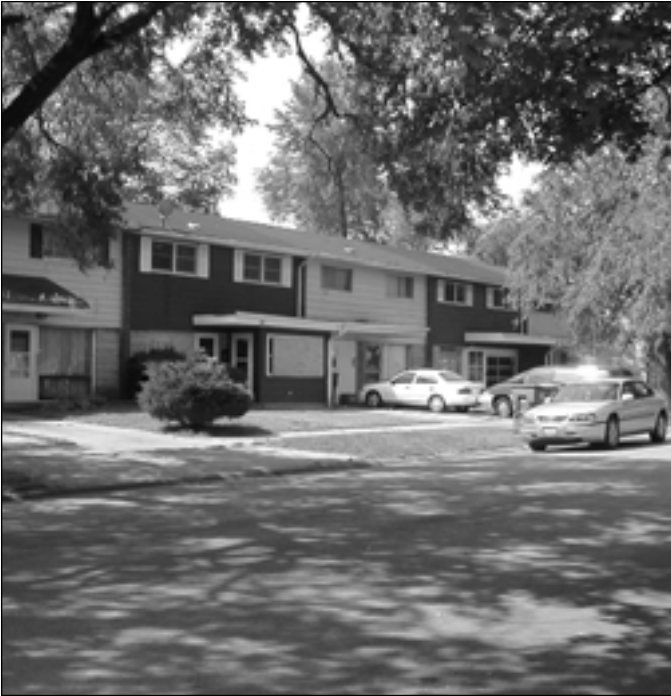
The physical conditions of Pacesetter are exacerbated by parking congestion, poor housing conditions and isolation from the rest of Riverdale.
