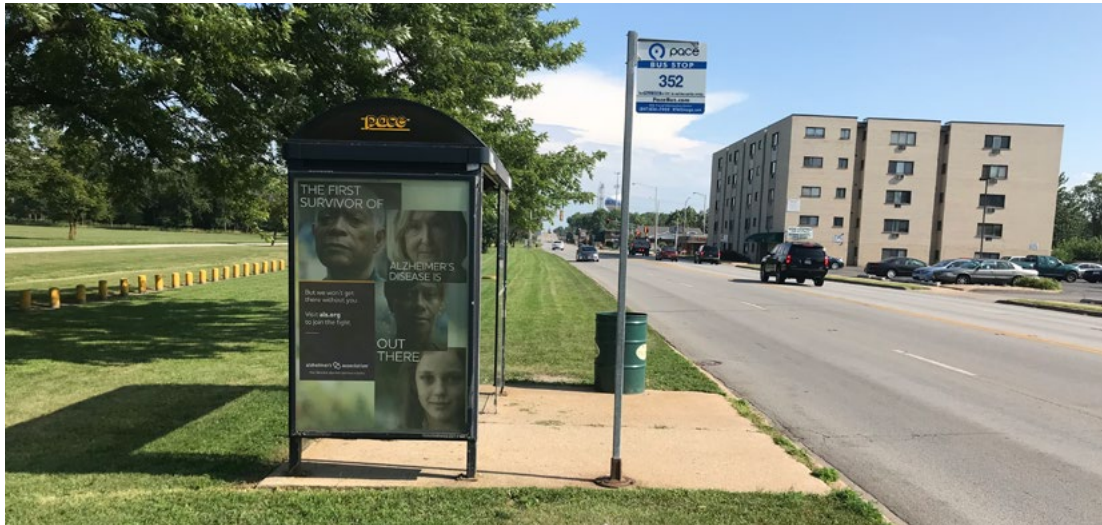
Figure 6. Pace bus stop without sidewalk access
