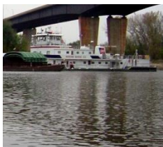
River Discharge 551,000 tons
